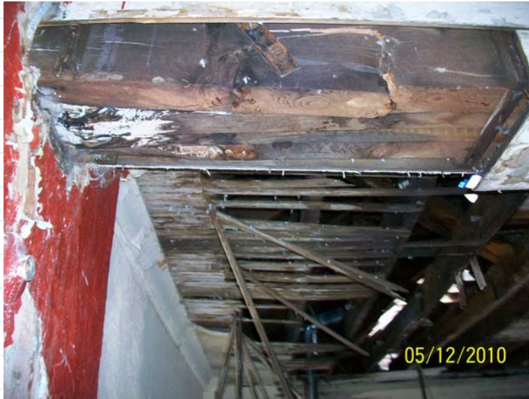
Truss #1, South Bearing
