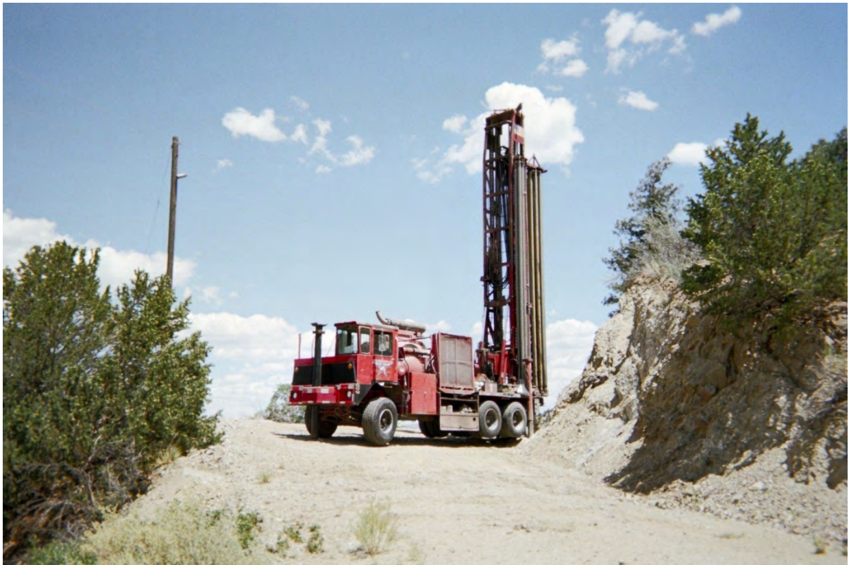
Drilling rig on Co 115 ready to drill PS-2d
