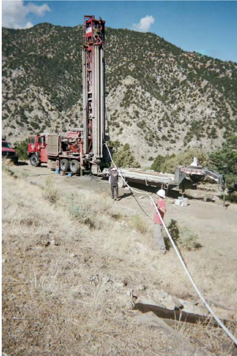
Drill crew feeding PVC pipe into drill hole PS-2c
