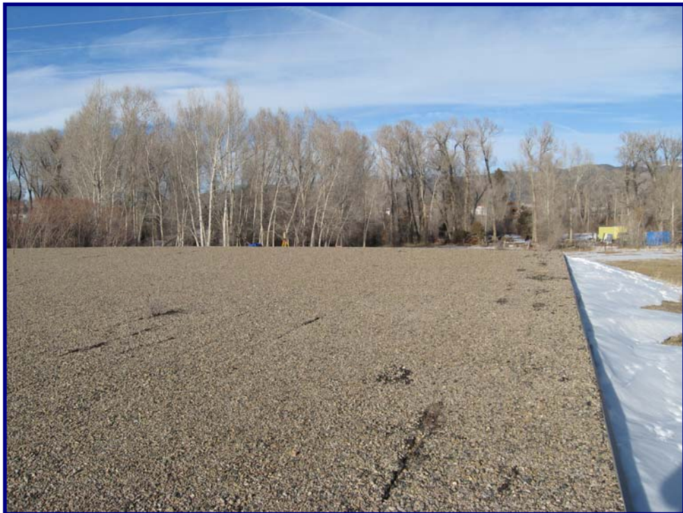
Photo 2 - Existing Built-Up Roofing Material
