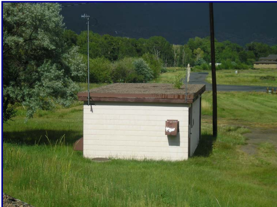
Photo 6 - Existing Water Treatment Building
