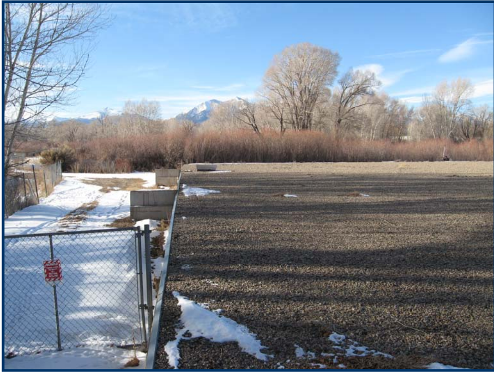
Photo 5 - Access hatch to be replaced
