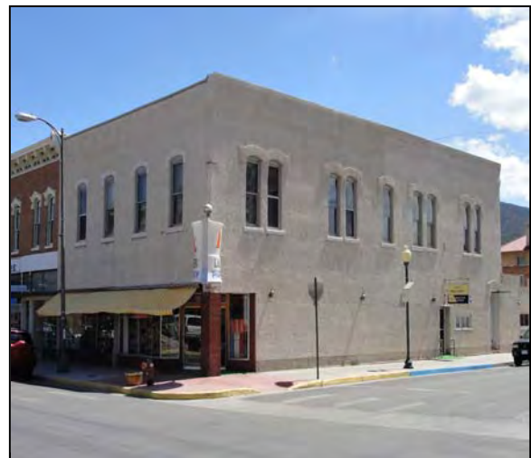
134-41 F Street, Davis/Thompson/Armstrong Drugs – The application of stucco to the exterior has covered up most historic materials and obscured many of the architectural details. In addition the storefront has undergone major alteration.
