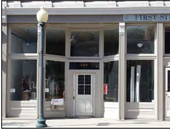
131-33 E. First St, Williams Grocery - This inset entrance has a transom and clerestories and a paneled door with stained glass.
