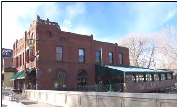
228 N. F St, Bon Ton Hotel, Manhattan Hotel – The addition on the rear and side can be differentiated as new rather than historic.
