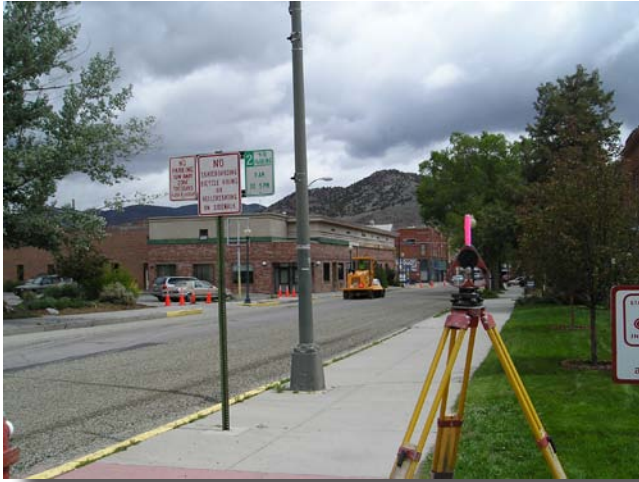
Chip seal project F Street
