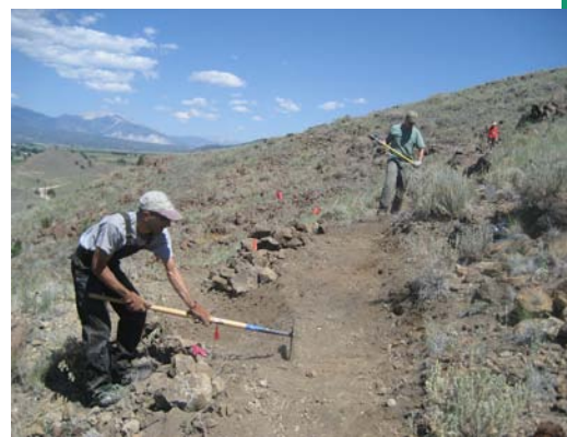
Salida Mountain Trails- Frontside Trail being built by local volunteers
