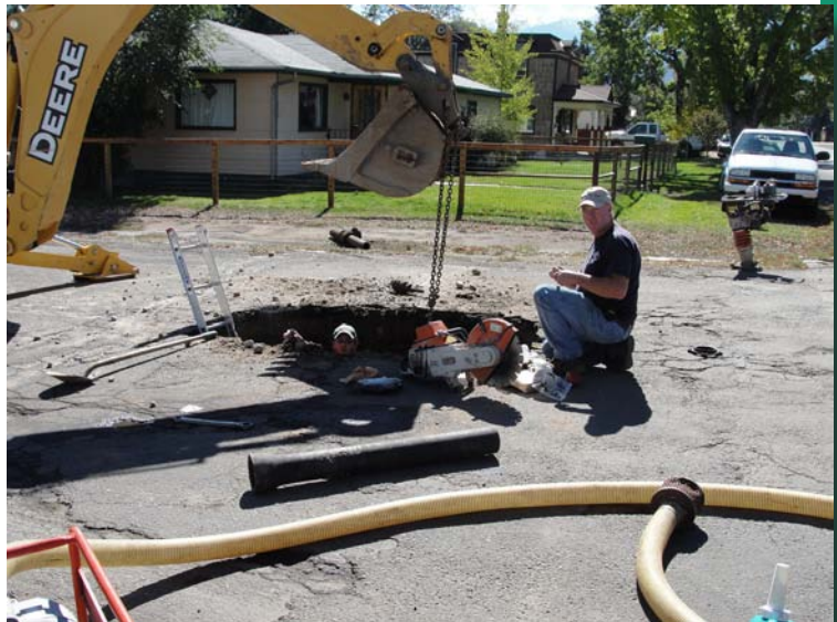
Public Works Repairing Water Lines
