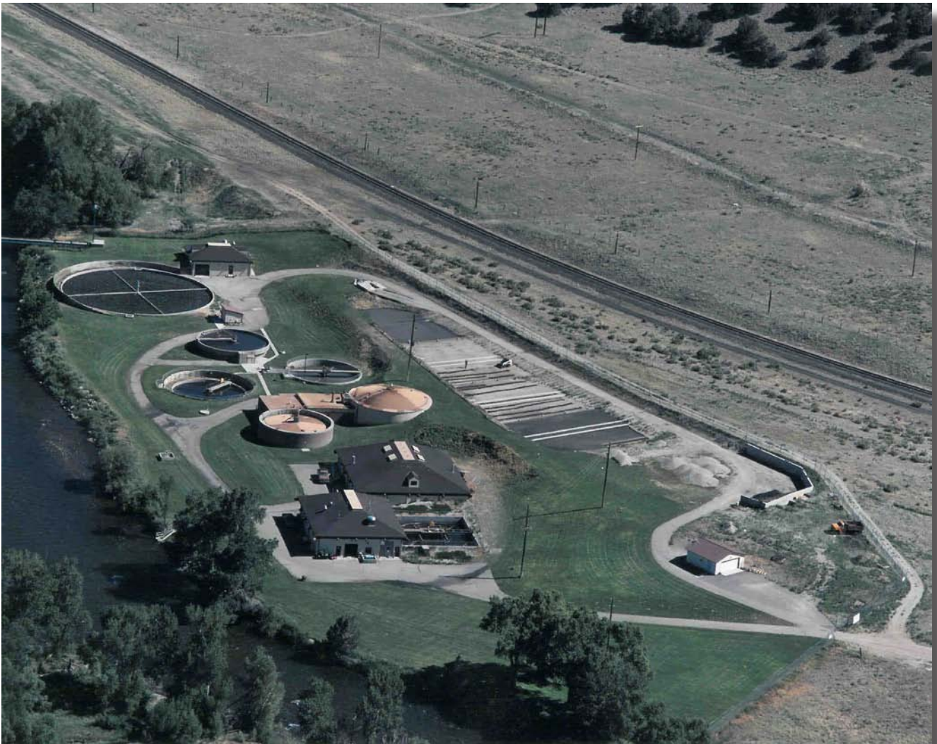
Wastewater Treatment Plant built in 1956 renovated in 1985
